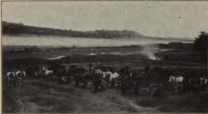
BUILDING THE LEVEE AT LAWRENCEBURG, IND., FOR THE PROTECTION OF THE CITY AGAINST FLOODS.
